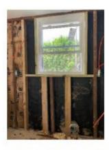
Photo 4: New window installed
