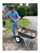
Photo 14: Mixing Concrete
