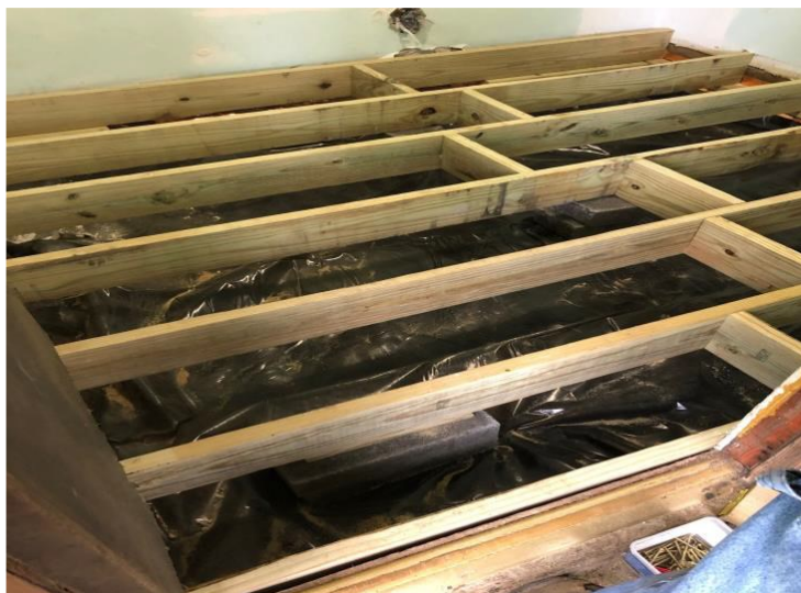
Picture 8: New Floor Joists/Plastic/Termite Guards
