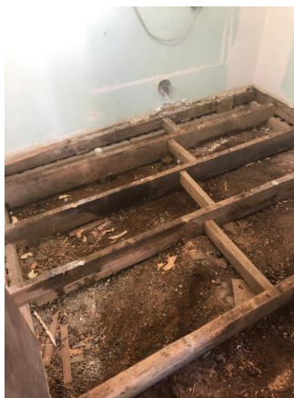
Picture 6: Faulty Floor Joists
